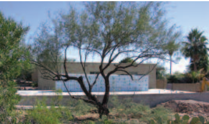
Sixteen stacks of Quad-Lock for the 1700ft addition.
