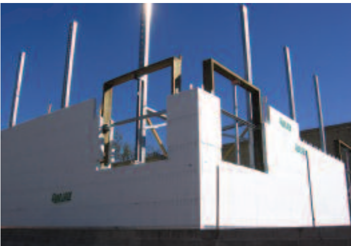
Day two of construction- installing the Quad-Lock panels.
